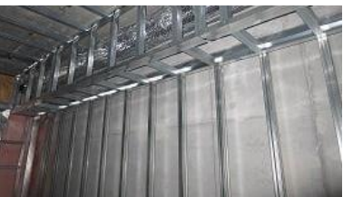
Metal (for plasterboard base: light steel frame)
