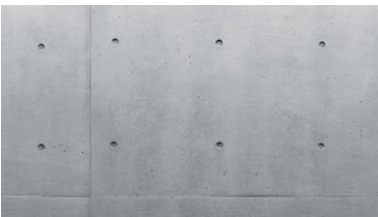
Concrete wall (with gypsum board substrate)
